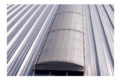
A number of proprietary barrel-vault systems are available. They are usually specified with Secret Fix Systems and for very low pitches. They can be used with single skin, built-up or composite roofs, with secret fix systems, curved roofs, flat roofs, along a ridge and in other low pitch applications.
