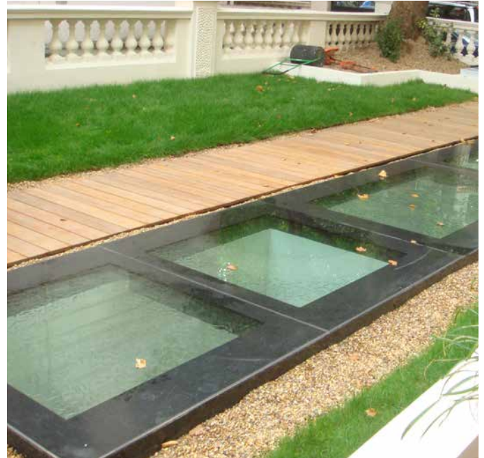
Garden area with walk-on rooflight over basement
