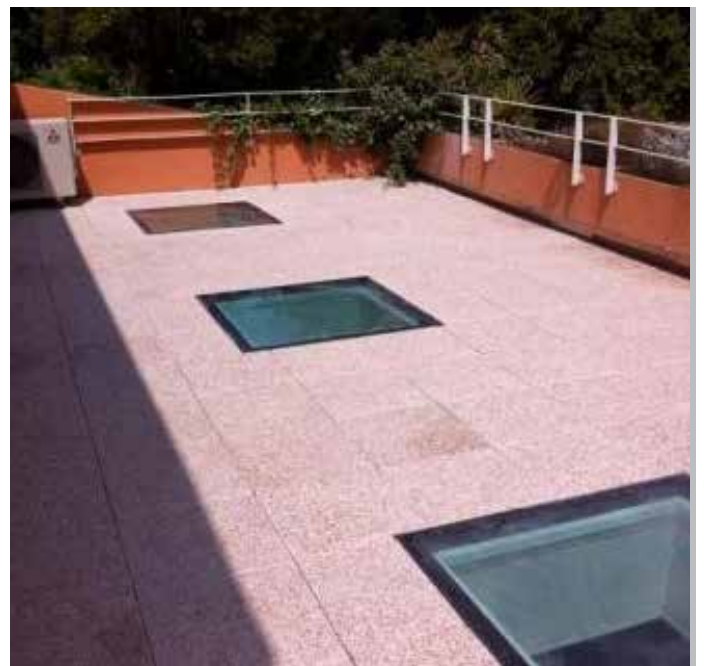
Roof terrace area
