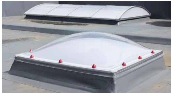
AFTER: Whitesales Em-Vault & Em-Dome polycarbonate rooflights provide excellent thermal insulation with high light transmission
