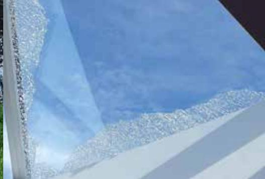
The glazing on this rooflight was not properly fixed, resulting in it being blown off in windy weather and ending up in a neighbour's garden. Luckily, no-one was injured in this instance.
